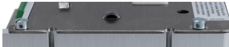
Figure 2-67: Sealing Screws Installed
