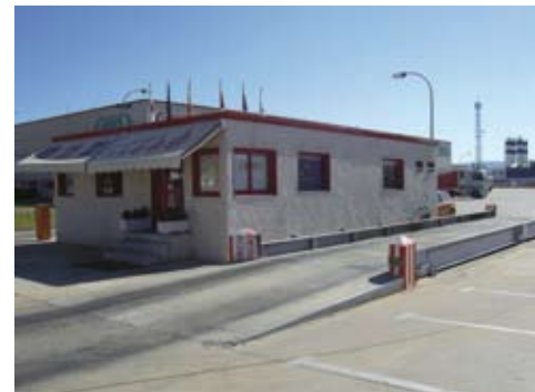
Vehicle scale for fast and precise accounting for incoming and outgoing goods
